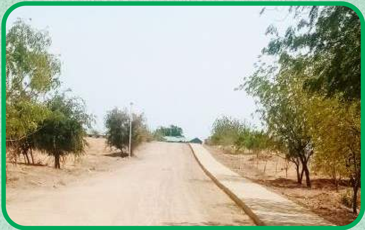
Construction of roads network at TUC
